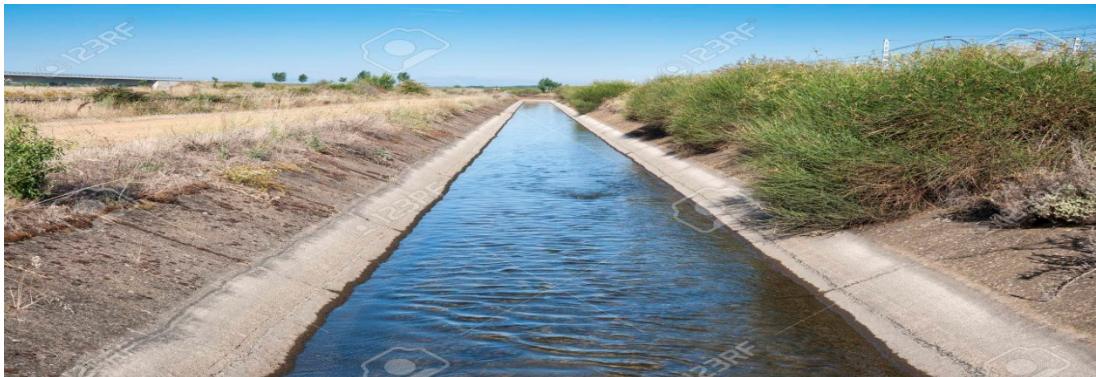
Figure 2: Concrete Channel with Trapezoidal Cross-Section for Agricultural Use
